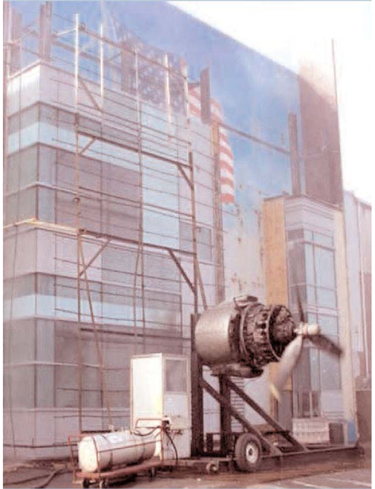
Figure 11. AAMA Dynamic Water Test
